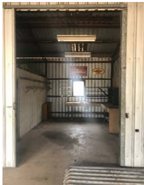
View of the garage / workshop area Inspected 06.02.18
