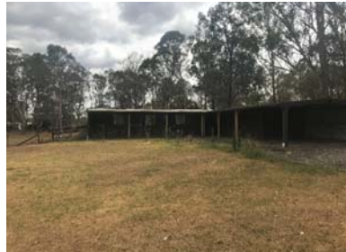
View of the carport & animal shelter Looking north Inspected 06.02.18
