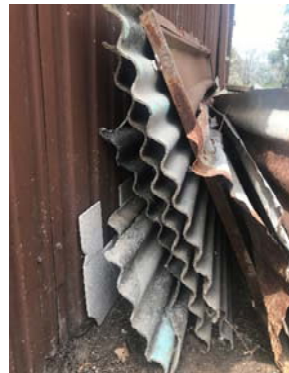
View of fibro cement sheeting adjacent to garage / workshop area Looking south Inspected 06.02.18
