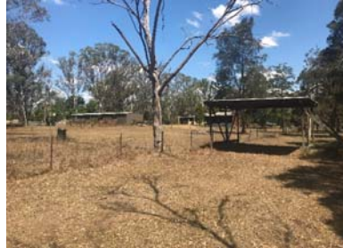
View of roof shelter and stockpile Looking south east Inspected 06.02.18
