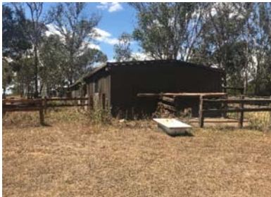
View of the animal shelter Looking east Inspected 06.02.18
