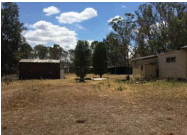
View of garage / workshop and house Looking north Inspected 06.02.18
