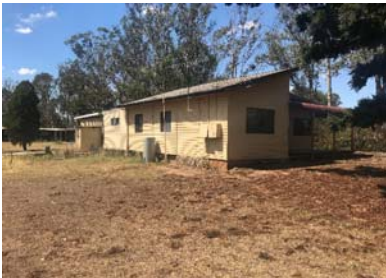
View of house Looking north east Inspected 06.02.18
